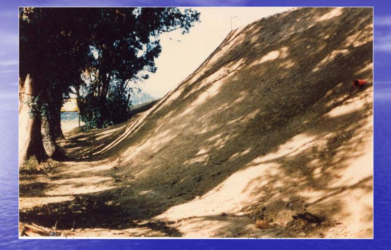
Example of a 45 degree fill face supporting a shopping center complex adjacent to a line of mature trees. The embankment was constructed using false layers of geotextiles spaced 1 foot apart (from Rogers, 1992)
