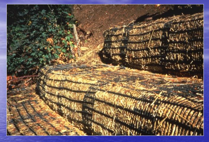
Geogrid-wrapped hay bales or gravel filled HDPE baskets can be used as facing elements for mechanically-stabilized embankments.
