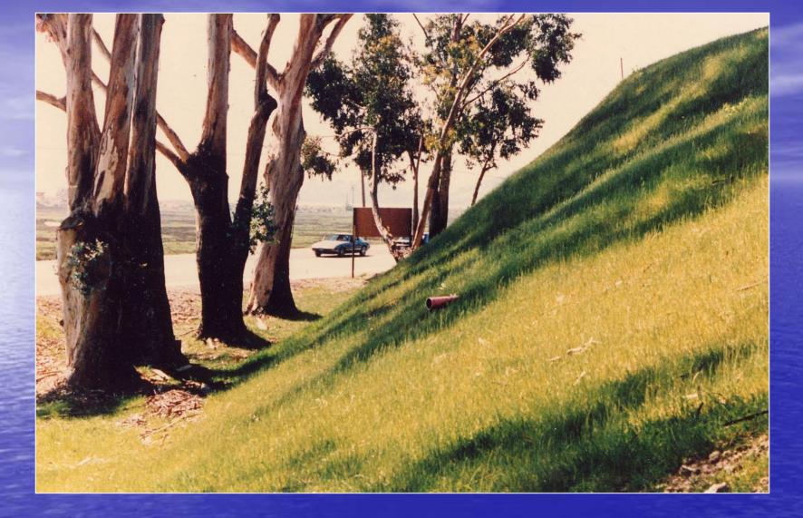
Same 45 degree fill slope after hydroseeding and sprouting of fescue grass mix (from Rogers, 1992). ENGINEERING FOR STORM SURGE AND WAVE ENERGY DISSIPATION
